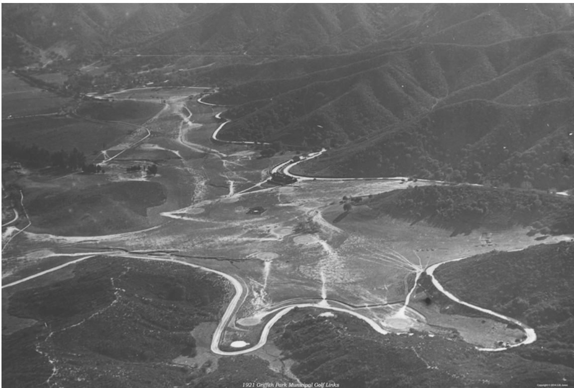
Looking south, at Municipal Links #1, towards Park Center
